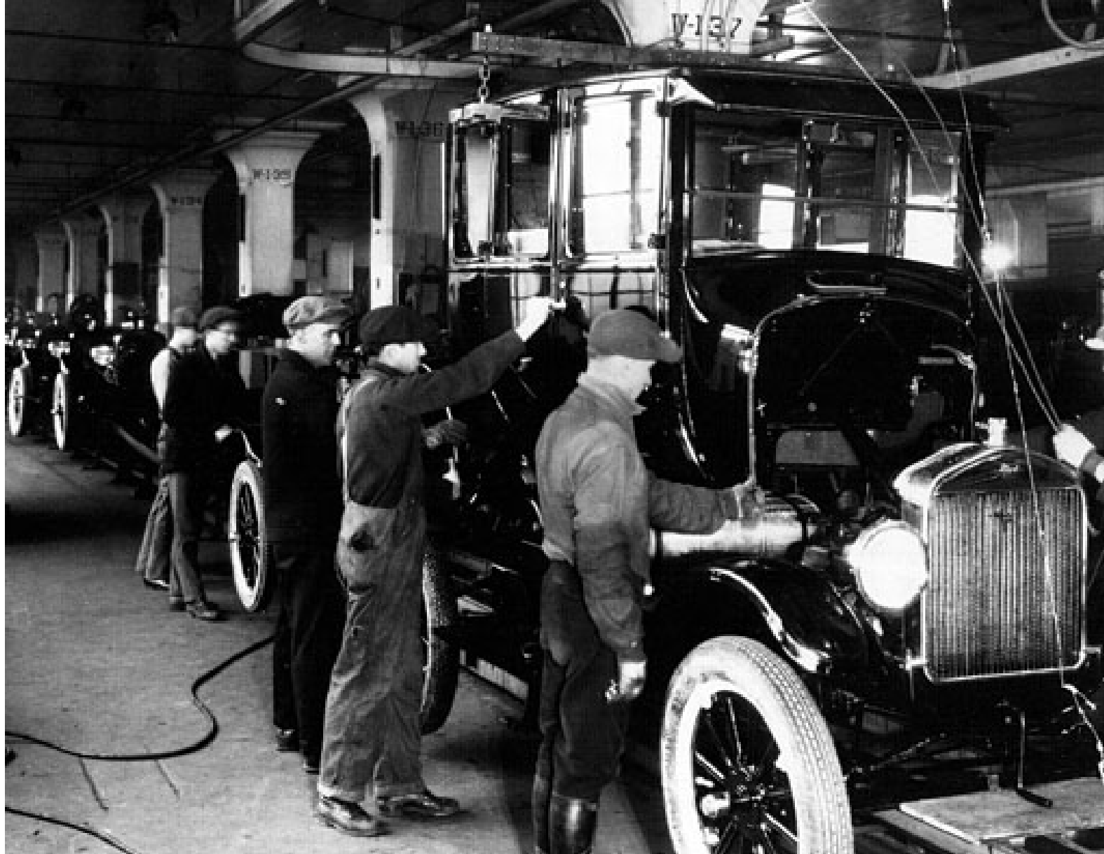
The body drop on the assembly line of the Highland Park Plant.
